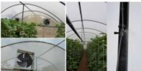
Fig. 4. Fan installation in the melon green house..
